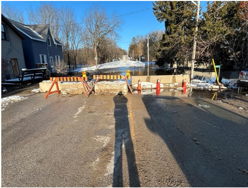
Barricades Installed Across Bruce Road 15 - March 15, 2026
