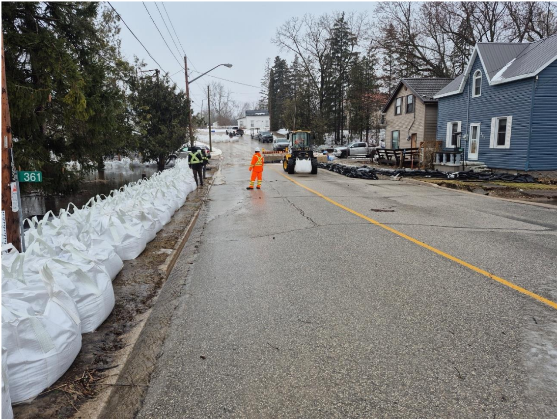
Temporary Cofferdam Installed - March 20, 2026
