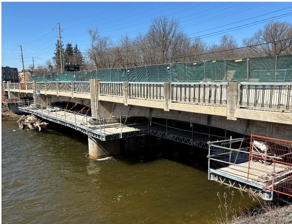
Photo above taken on April 17 th , 2025. (East (span 3) Suspended Platform Reinstatement In Progress)
