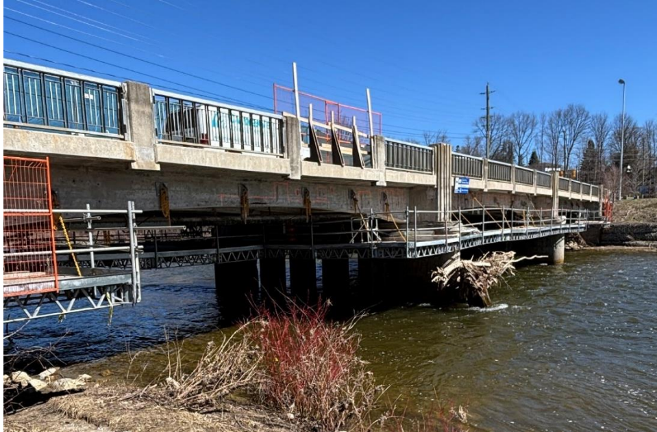
Photo above taken on April 17 th , 2025. (West (span 1) Suspended Platform Reinstatement In Progress)
