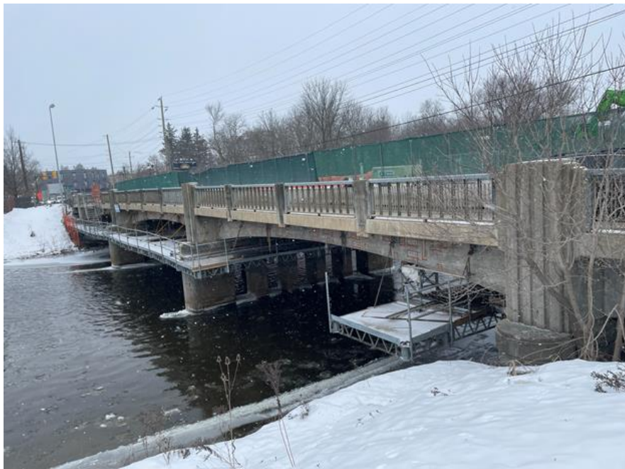
Photo above taken on December 23 rd , 2024 (East (span 3) Suspended Platform Removed)
