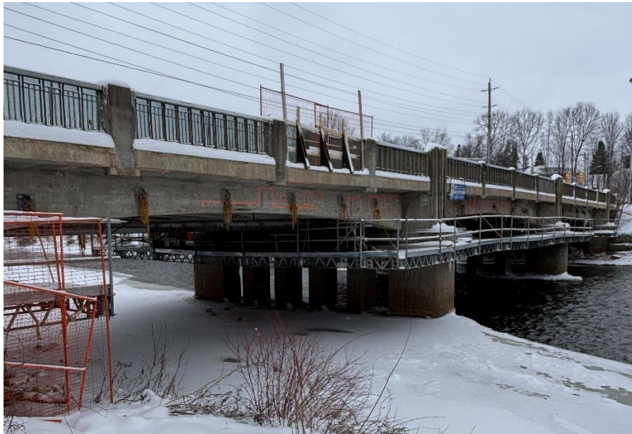
Photo above taken on January 13 th , 2025. (West (span 1) Suspended Platform Removed)
