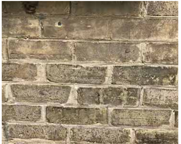
15a 254 High Street, intact historic brickwork and intact lime mortar and tuck pointing
