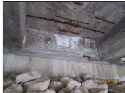
EXPOSED SOFFIT REINFORCEMENT
