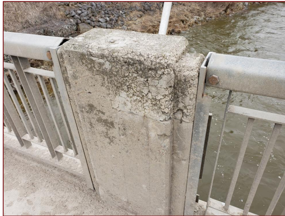
Image 29: Concrete Railing Post Deterioration North Side - Three
