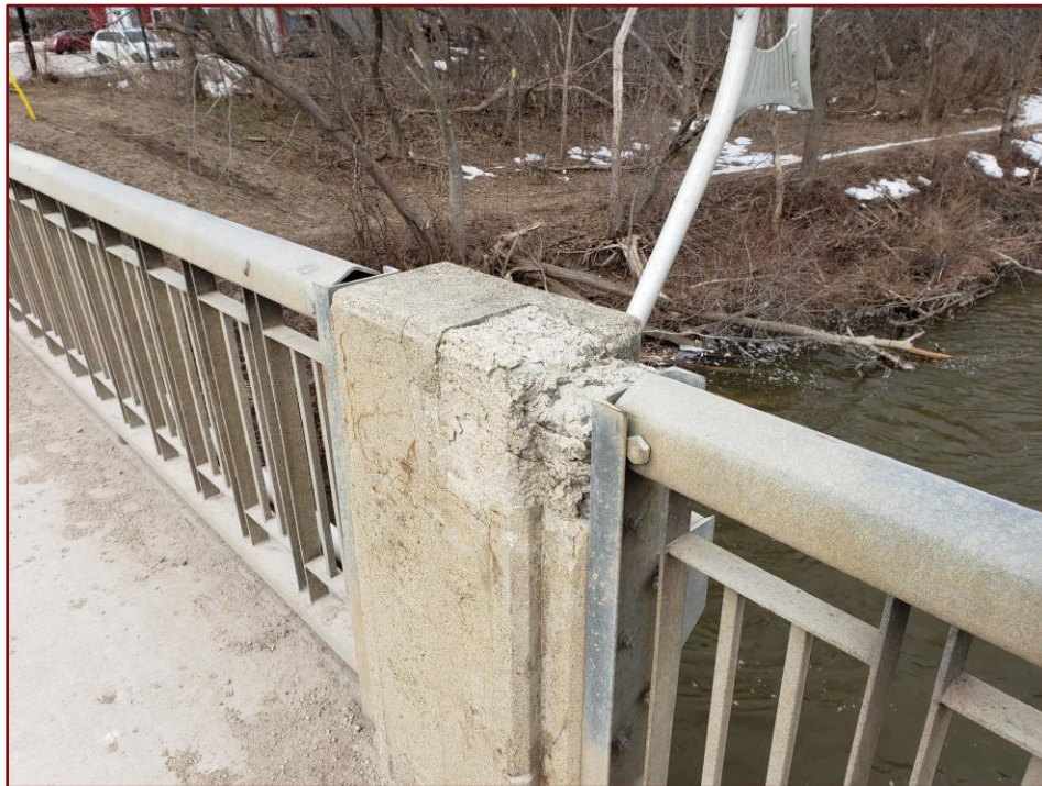
Image 29: Concrete Railing Post Deterioration North Side - Three
