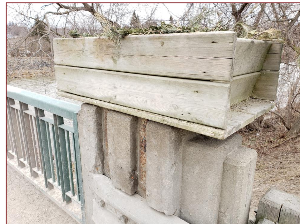
Image 25: Planters Box in Former Light Standard Location on Top of Stanchion
