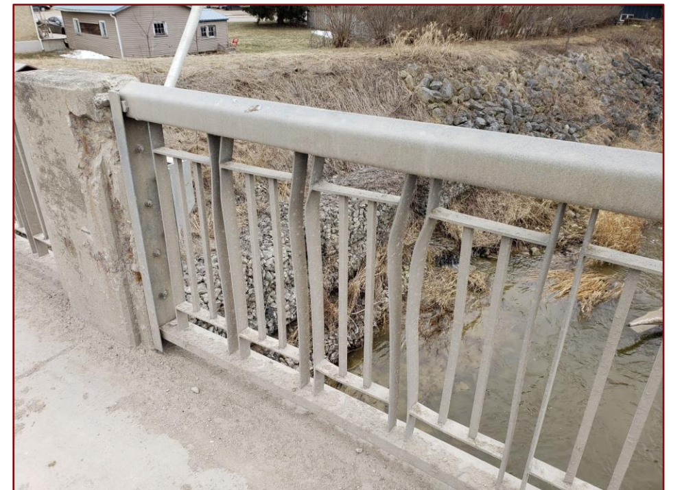
Image 31: Railing Damage Southeast Side
