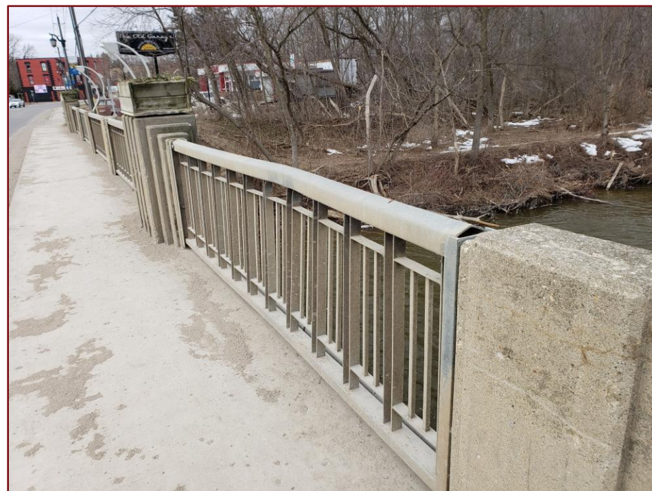
Image 33: Railing Impact Damage North Side
