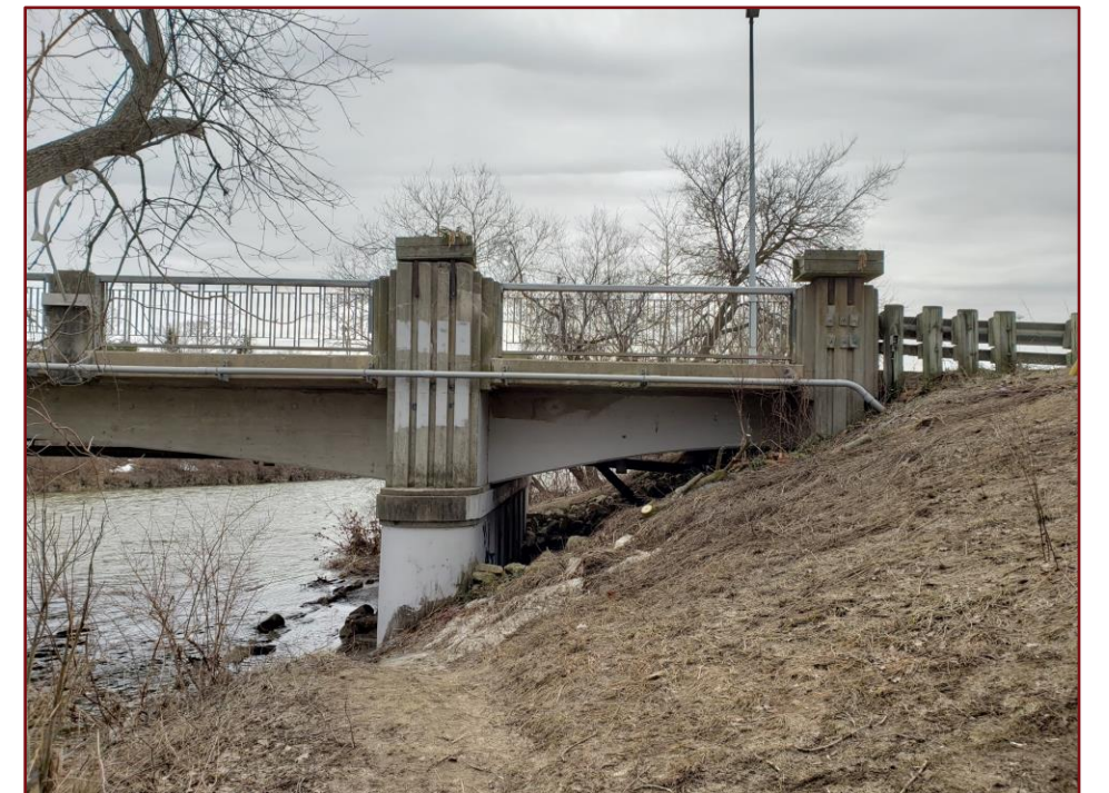
Image 19: Short Cantilevered West Approach Span
