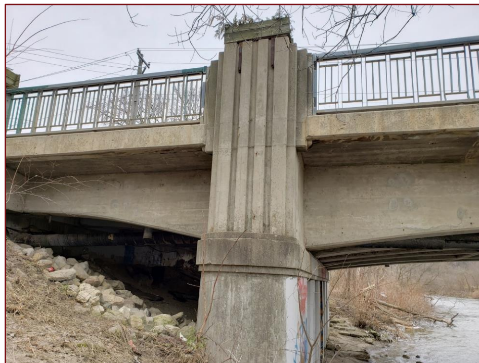
Image 23: Interior View of Stanchion/Pillar with Embossed Detailing
