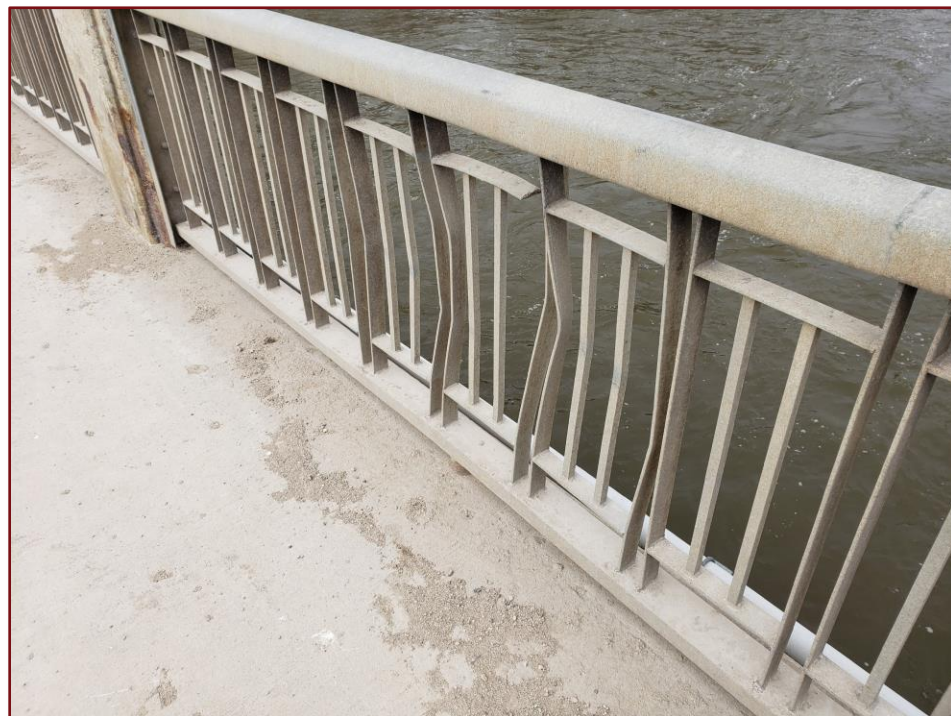
Image 33: Railing Impact Damage North Side
