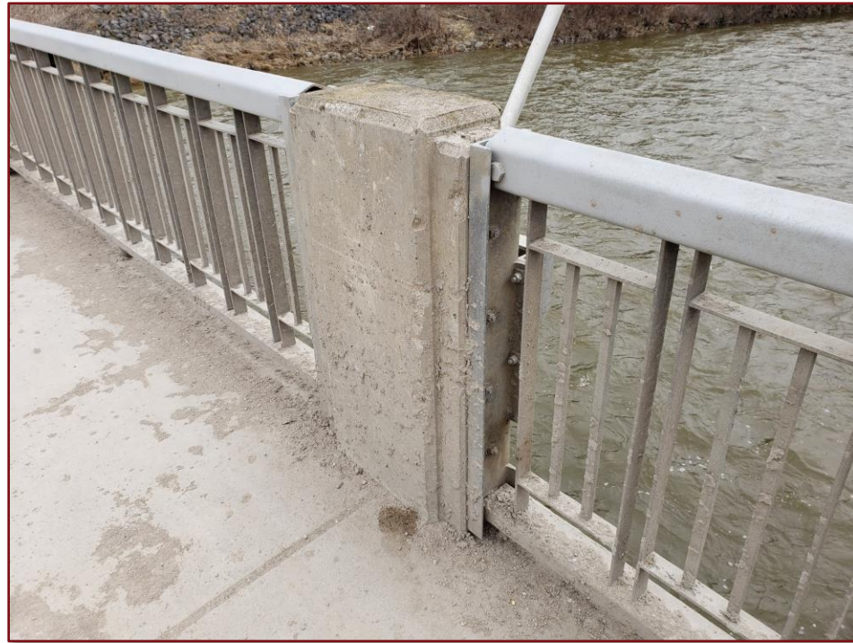
Image 27: Concrete Railing Post Deterioration North Side - One
