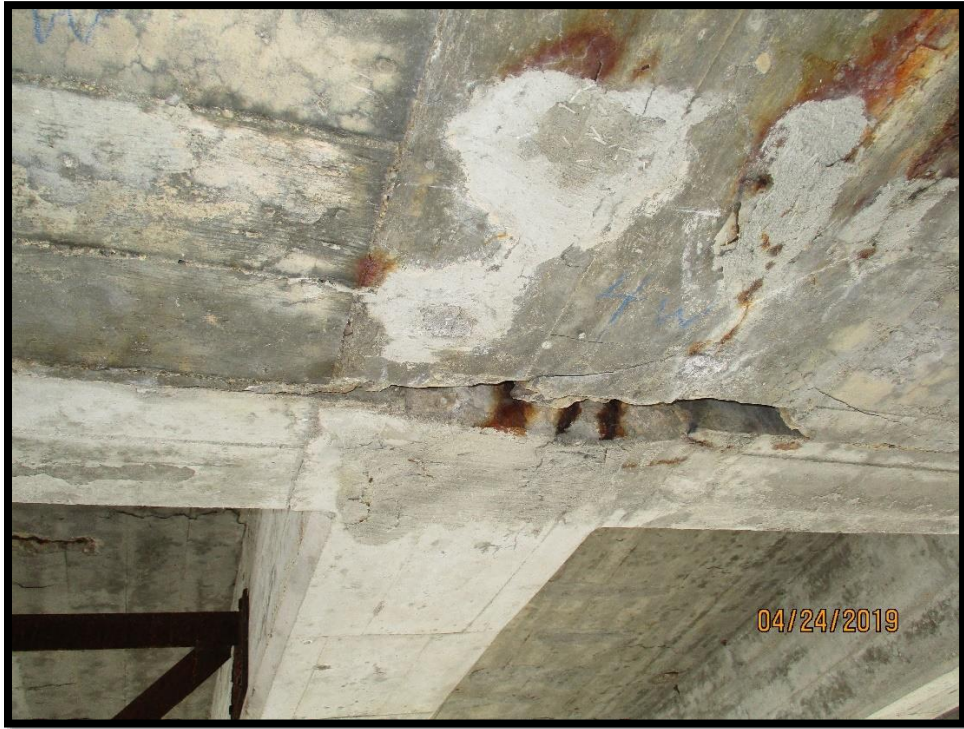
Typical pop-outs, corner spall from insufficient cover
