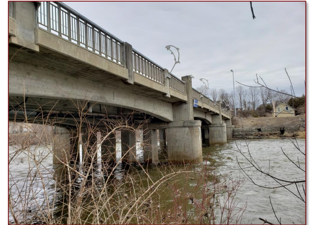
Image 19: Short Cantilevered West Approach Span
