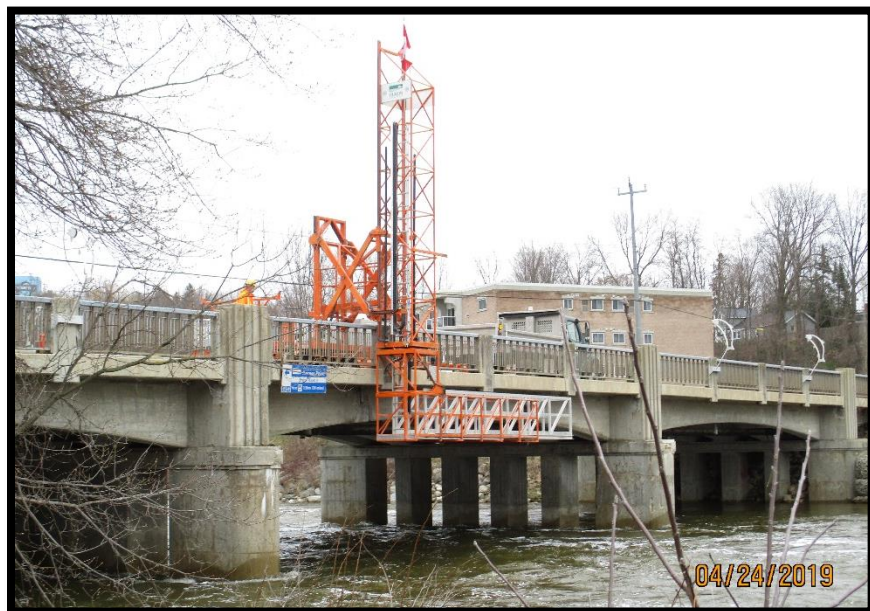
Access platform before turning under bridge deck
