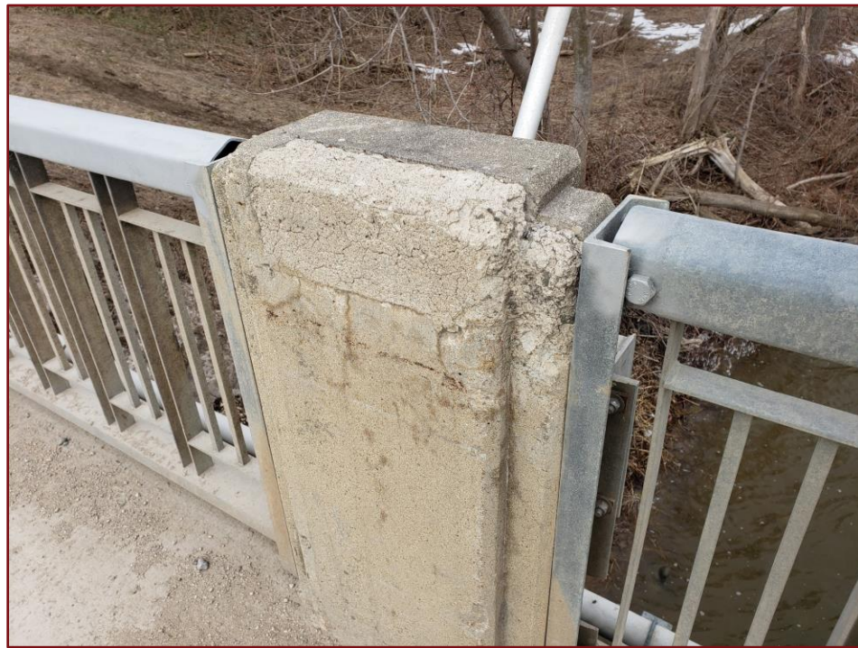
Image 27: Concrete Railing Post Deterioration North Side - One
