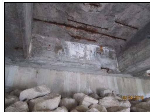
EXPOSED SOFFIT REINFORCEMENT
