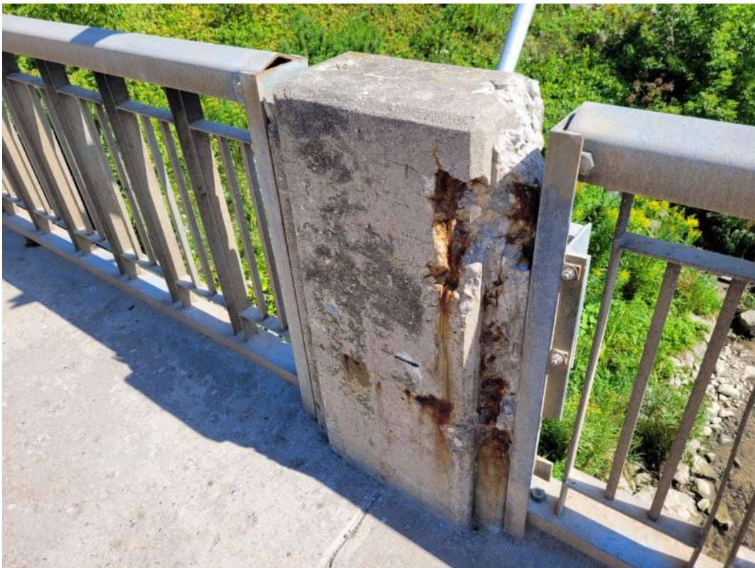
6-South Railing Spall
