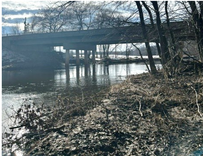
Figure 6: Bridge over the Teeswater River on Bruce Road 20
