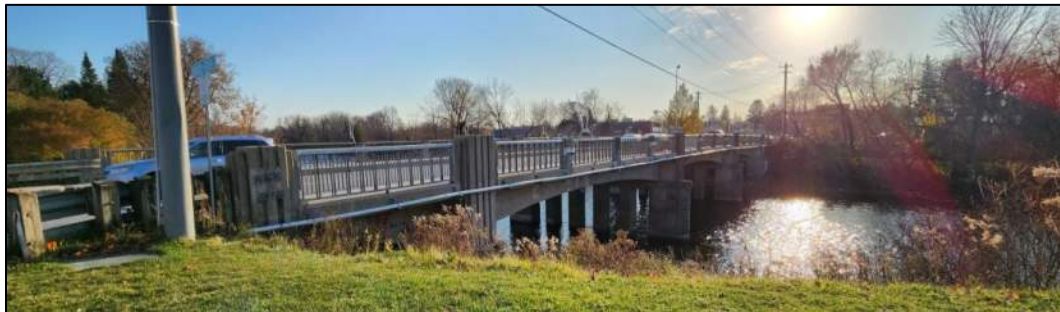
Photo 1: North Elevation of Structure 0419550, Walkerton, Ontario
