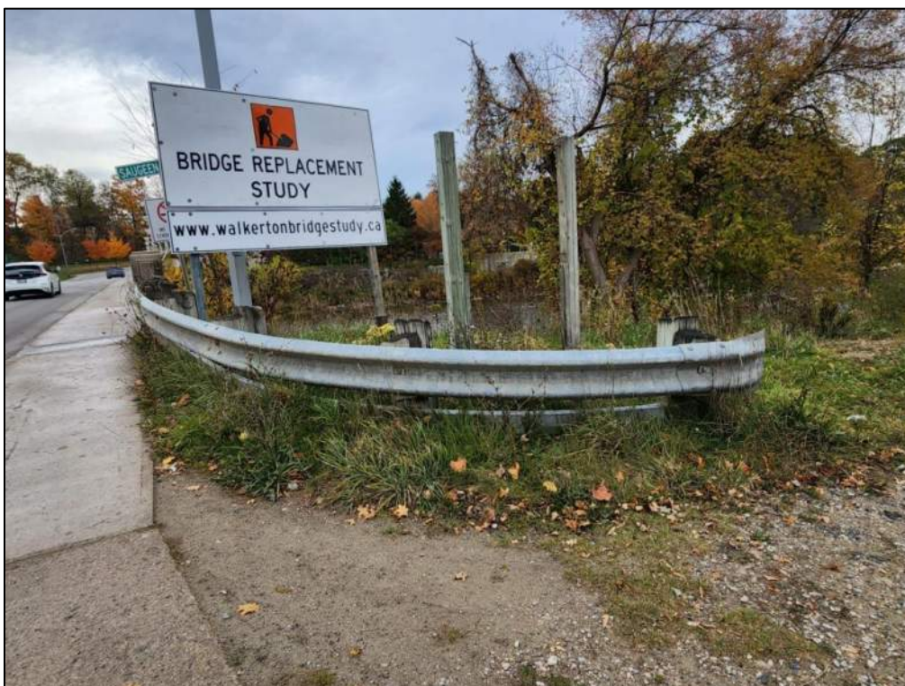
Photo P34 – South-West Guiderail (good condition – splits on wooden posts)
