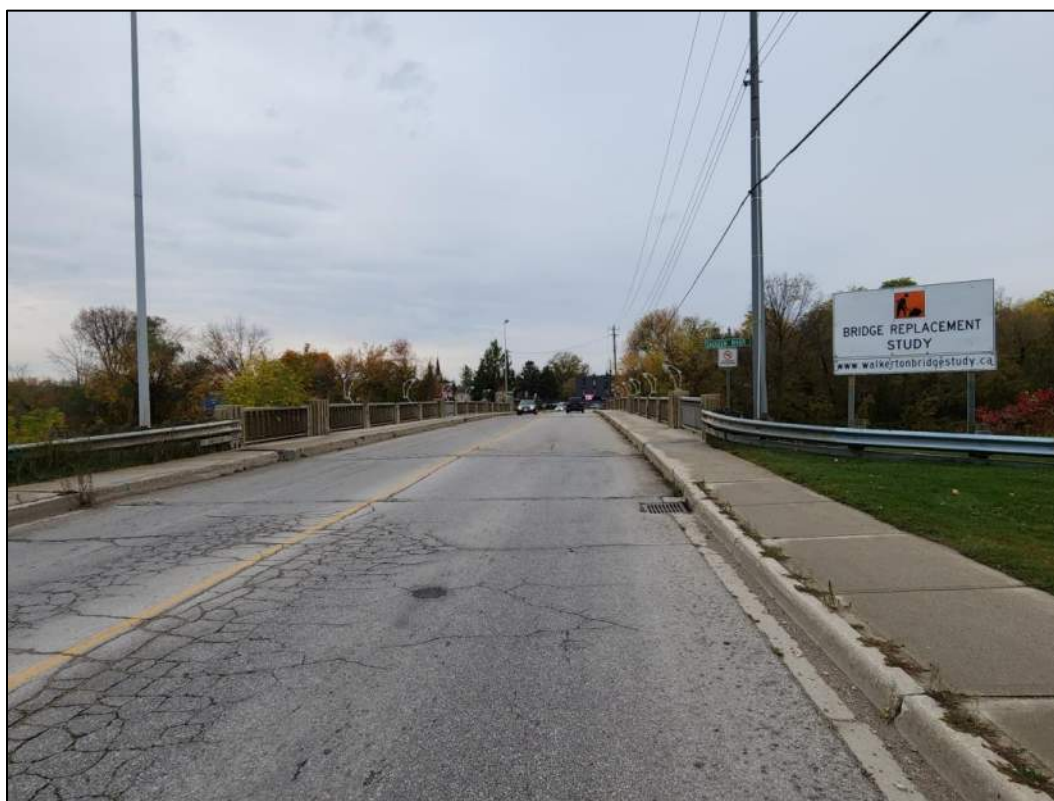
Photo P4 – General Overview of Deck, looking West
