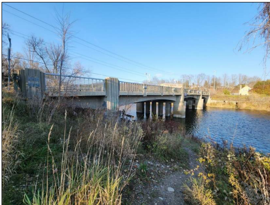
Photo P2 – South Elevation
