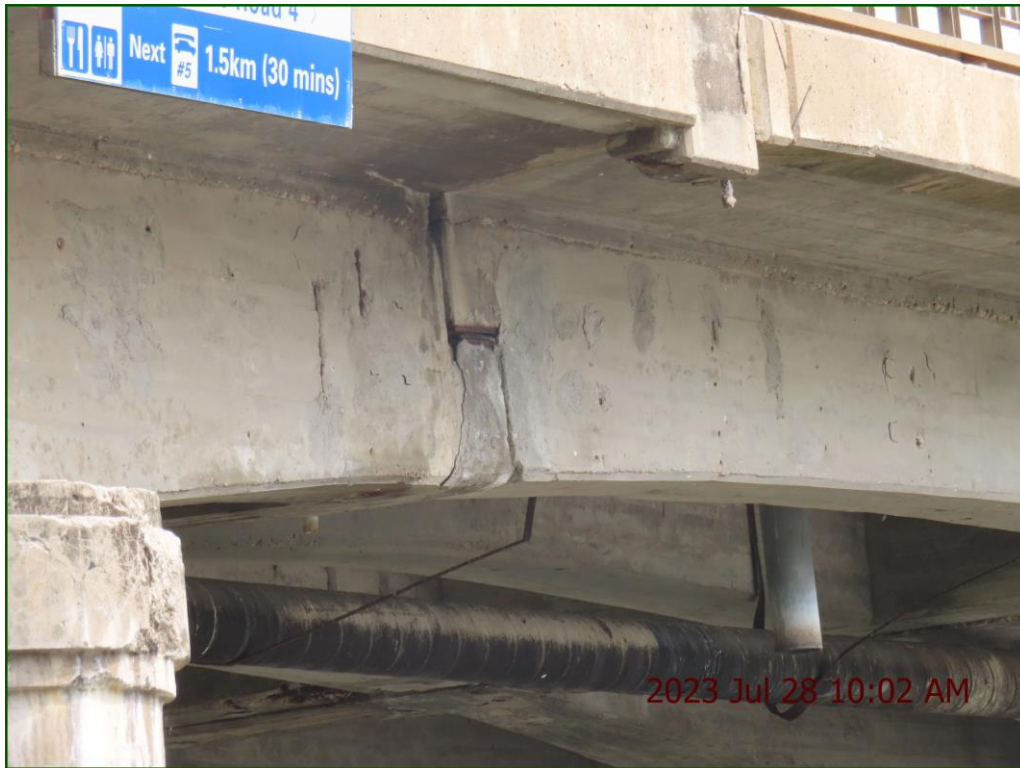
Description: Girders: Mid-span Joint
