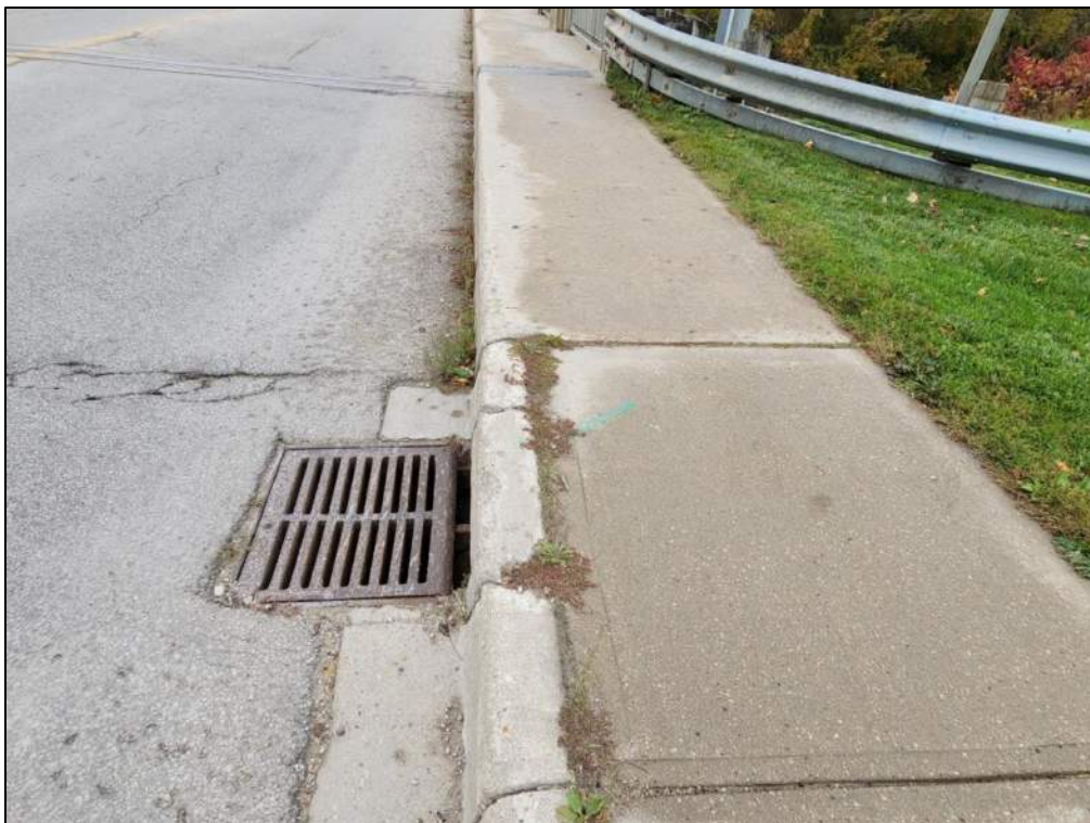
Photo P35 – North-East Catch Basin
