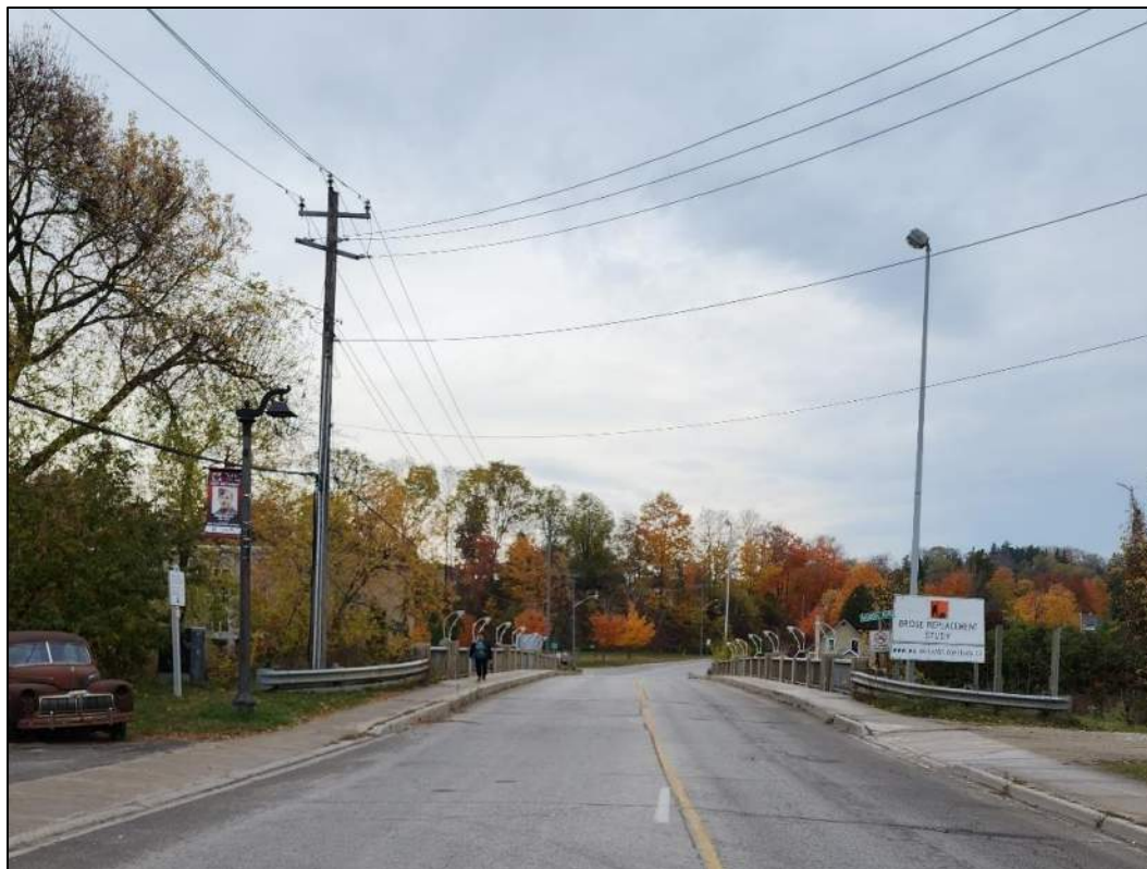
Photo P3 – General Overview of Deck, looking East
