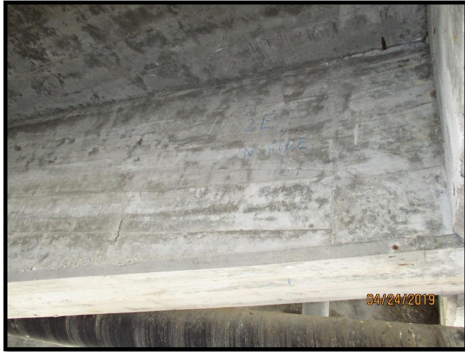
Typical cantilever beam face in good condition
