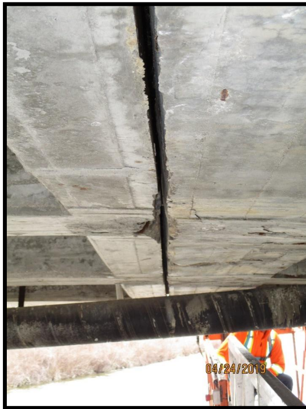
Soffit of west joint
