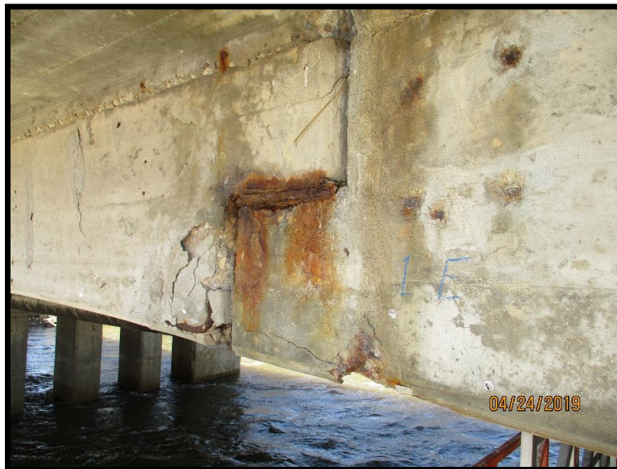
Elevation of connection showing support corbel on the right and dapped end of beam on the left
