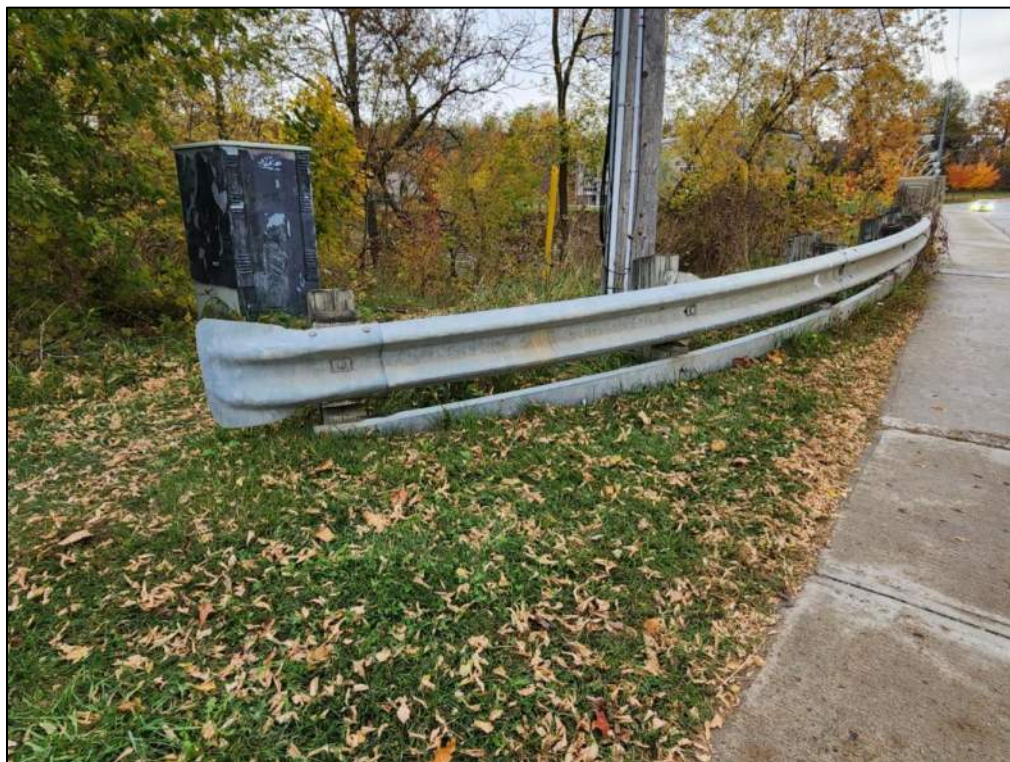
Photo P32 – North-West Guiderail (good condition – splits and rot on wooden posts)
