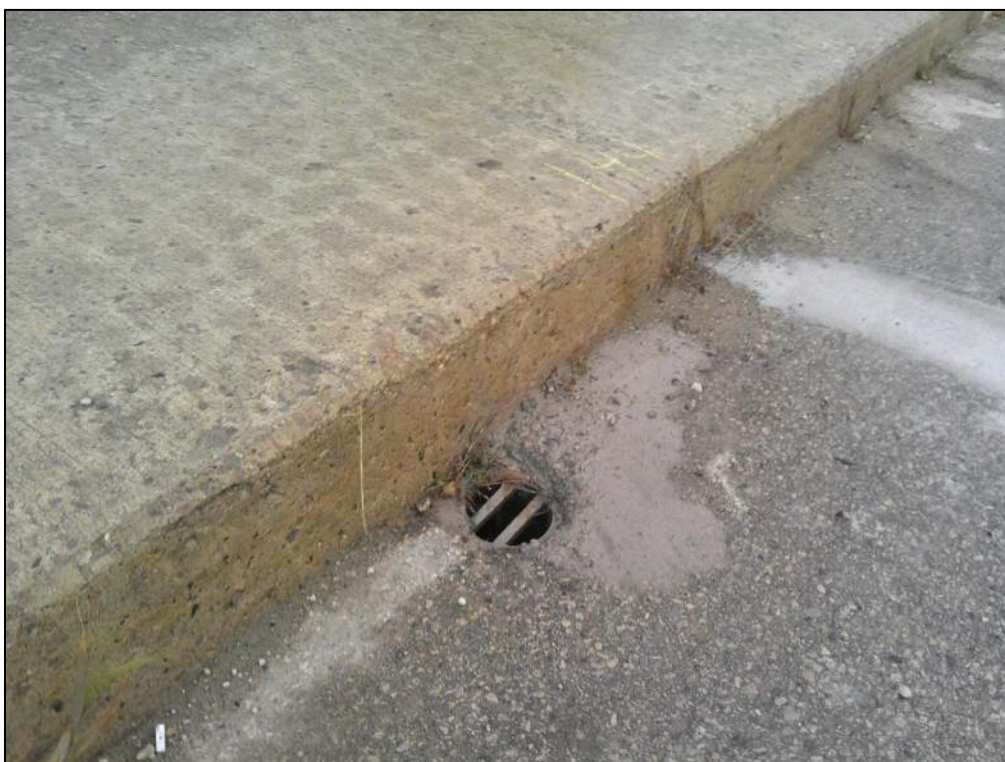
Photo P36 – Deck Drains – Typical
