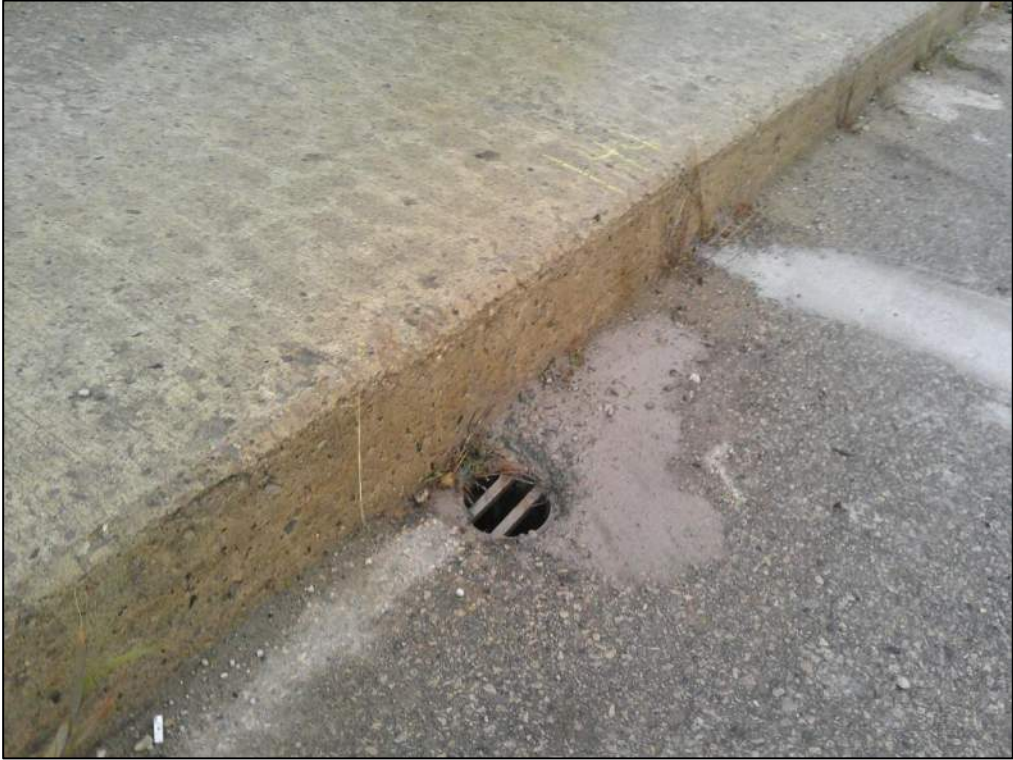
Deck Drains – Typical
