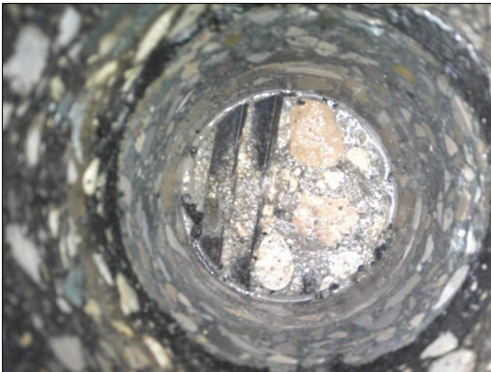
Photo P95 – Inside Core C12 (square rebar-good condition)
