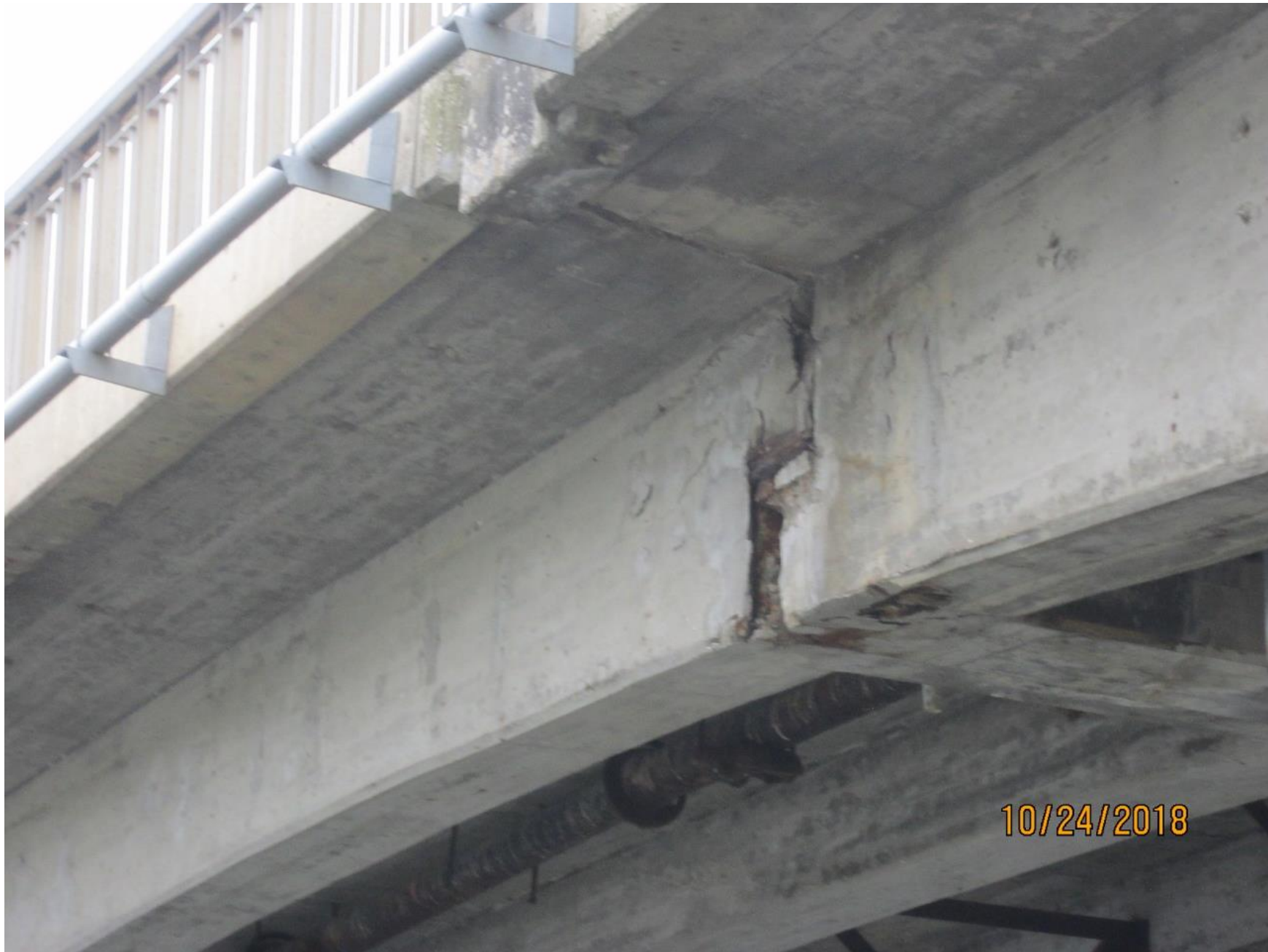
West Beam Joint
