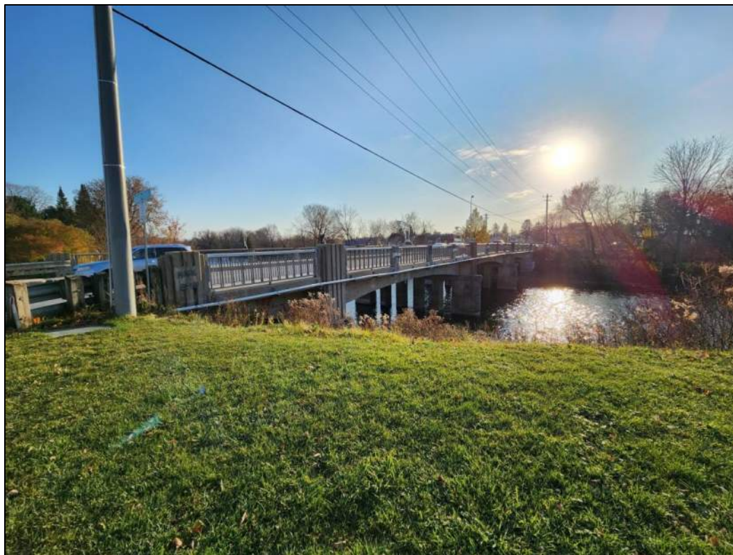
Photo P1 – North Elevation
