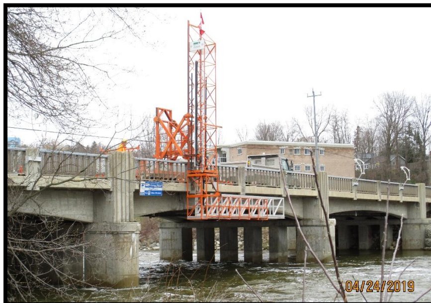
Access platform before turning under bridge deck
