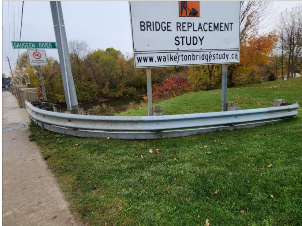
Photo P31 – North-East Guiderail (good condition – splits on wooden posts)
