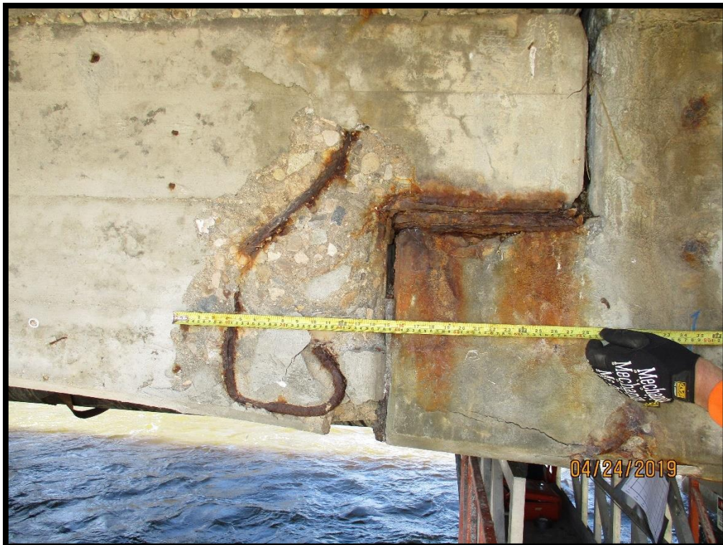
South exterior beam face – after scaling loose concrete
