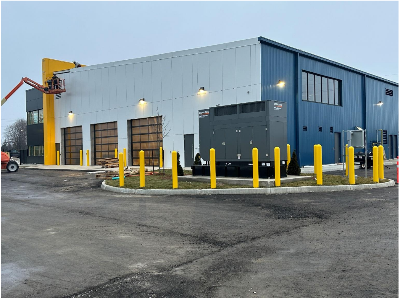
Roof flashing completed and bollard covers installed on February 1, 2024.
