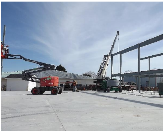
Erection of Structural Steel.
