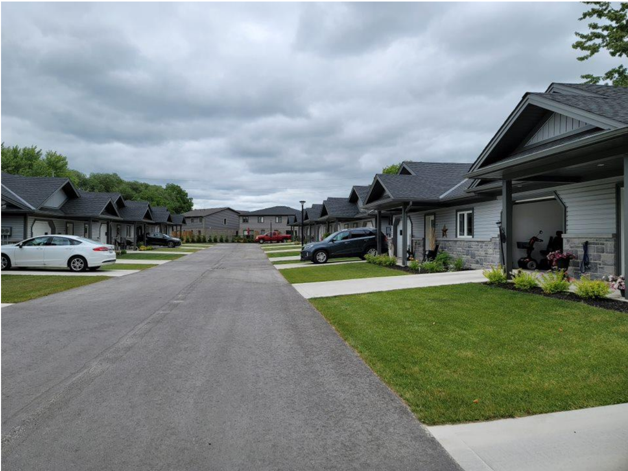
Townhouses recently completed in Walkerton
