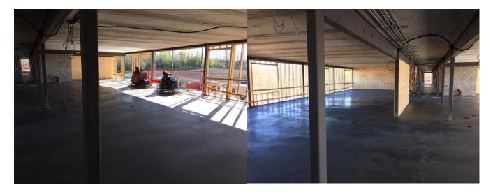
In late May, wood roof trusses were installed in the sloped roof section of the building, which completed the majority of the building's structure. The flat roof section of the building was previously installed using precast concrete slabs which is the same as the building's floor systems.
