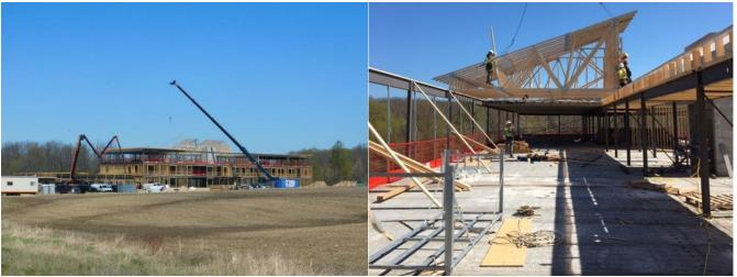
Throughout April, May and June, work on framing interior partitions and loadbearing walls has been underway. The office floor slab was poured first so framing in that area is now complete. Wiring and sound batt is being installed within the wall cavity and will be ready for sheeting in the near future.
