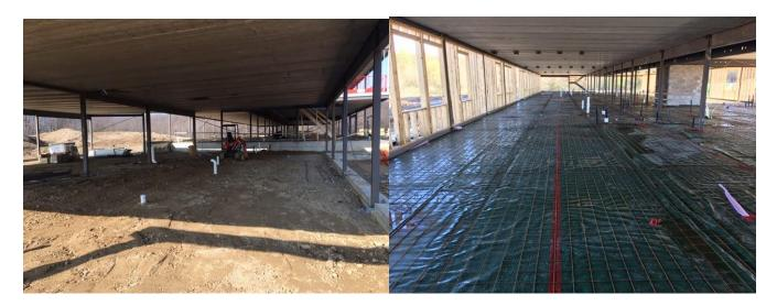
During April and May, the concrete floor slabs were poured on the ground floor in the apartment and office areas of the building. As soon as these slabs were complete, work was able to start on the ground floor for framing both the interior and exterior walls.
