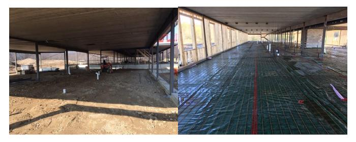
During April and May, the concrete floor slabs were poured on the ground floor in the apartment and office areas of the building. As soon as these slabs were complete, work was able to start on the ground floor for framing both the interior and exterior walls.
