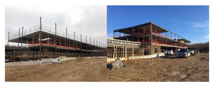
During April and May, underground services were installed throughout the building in preparation for the pouring of the floor slabs in both the apartment and office. Services such as electrical and plumbing were placed under the slab.
